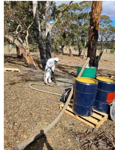
Vacuuming the Ash into Drums
